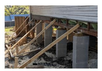
Advantages: Pier and beam foundations offer easy access to utilities and are more flexible in areas with unstable soil.
